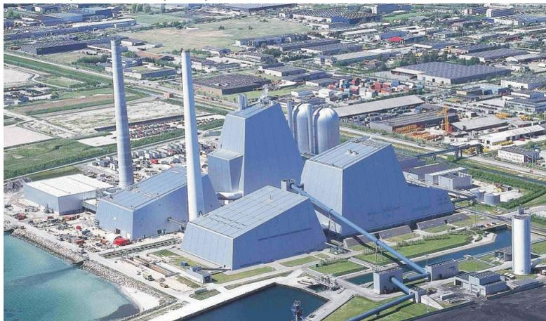
Avedøre Unit 2 (AV2), commissioned in 2001 and owned by Dong Energy, is one of the most efficient, fuel flexible, and environmentally friendly power plants in the world. In addition to generating electricity, the plant also supplies heat to the Copenhagen district heating network. The main plant of AV2 is an Ultra Super Critical (USC) boiler supplied by BWE.
