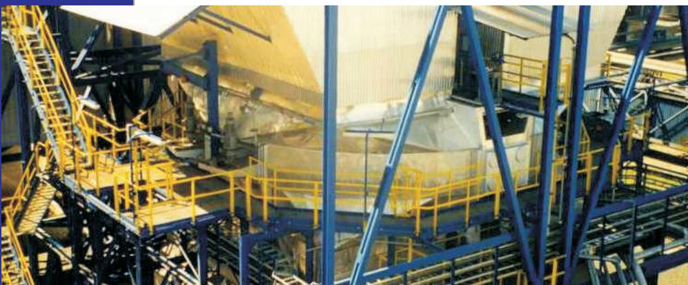
As the untreated flue gas is very aggressive due to high content of SO<sub>2</sub>, SO<sub>3</sub>, HF and dust, the heating elements are protected with enamel as corrosion protection.
