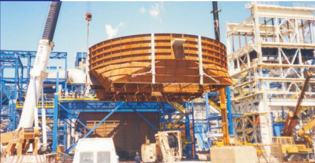
In 1998 BWE was awarded contract from STF S.p.A., Italy for the delivery of a Gas-Gas Heater (GGH) for installation in a new deNOx "Tail-end" plant. This plant cleans the flue gases from a coal-fired power station at the Enel owned Sulcis Power Station at Porto Scuso, Sardinia, Italy.
