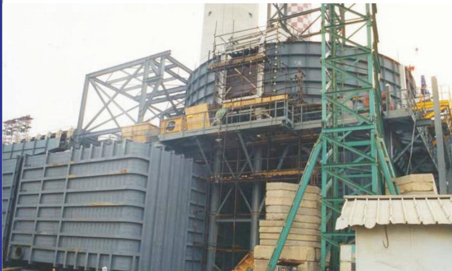
In 1997 BWE was awarded contract from Snamprogetti, Italy for the delivery of a Gas-Gas Heater (GGH) for installation in a new combined deSO<sub>x</sub> and deNO<sub>x</sub> plant a so-called SNOX plant. This plant cleans the flue gases from a coke-fired power station at the Agip Petroli owned Gela refinery at the south coast of Sicily.
