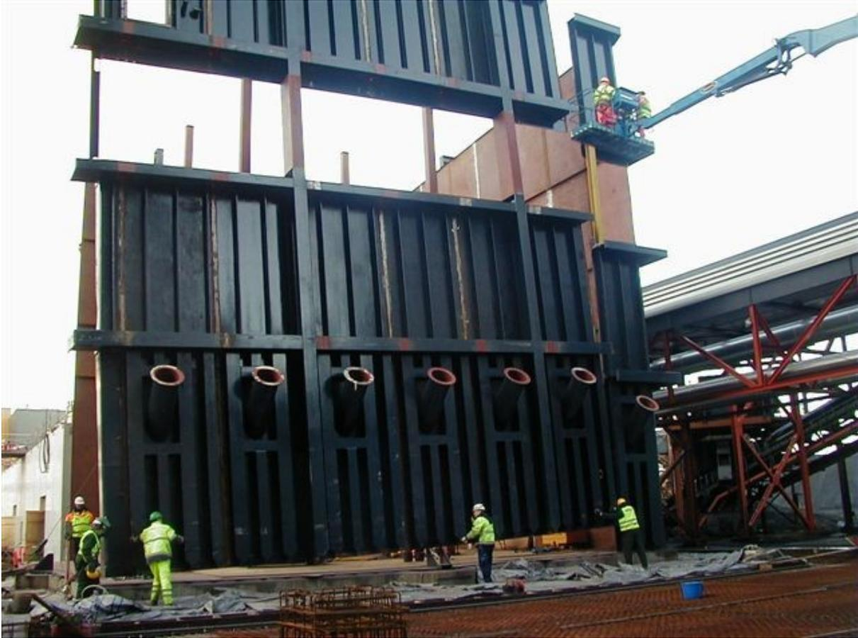
*Figure 7 The third JBR wall is lifted into place on January 26, 2009*
