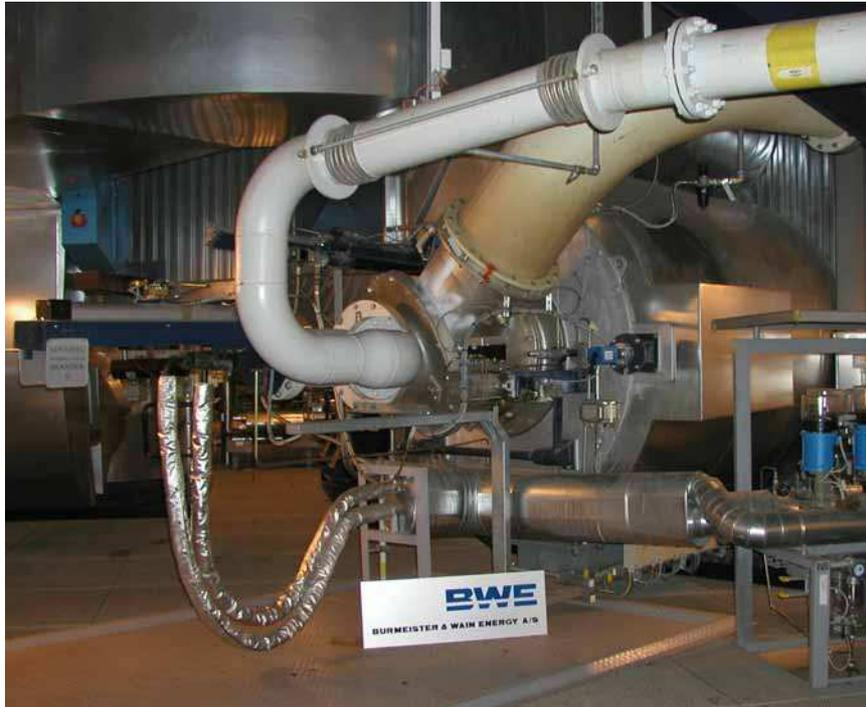
**Figure 14.** Multi fuel circular burner for tangential firing at AVV2.
