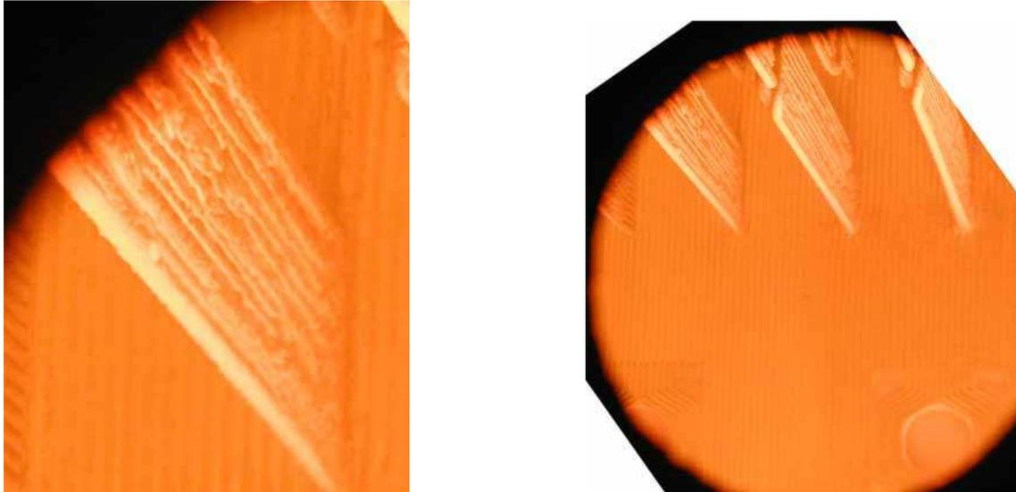
**Figure 15.** Superheater bundles above the furnace showing deposits from wood PF fuel.
