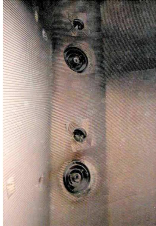
**Figure 3.** Openings for burners and over burner air in a furnace corner.
